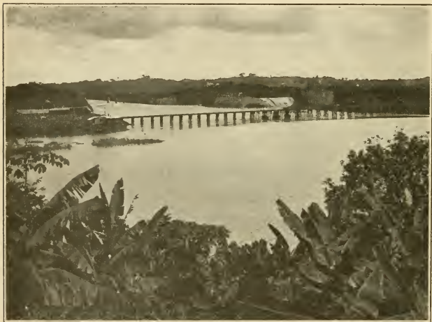
FIG. 2. GATUN SPILLWAY. LAKE DISCHARGING OVER SITE OF DAM AND THROUGH CHANNEL.
